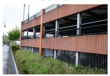
Note the railings on the ground floor. Similar railings should be put along this edge of the second floor to prevent access.
